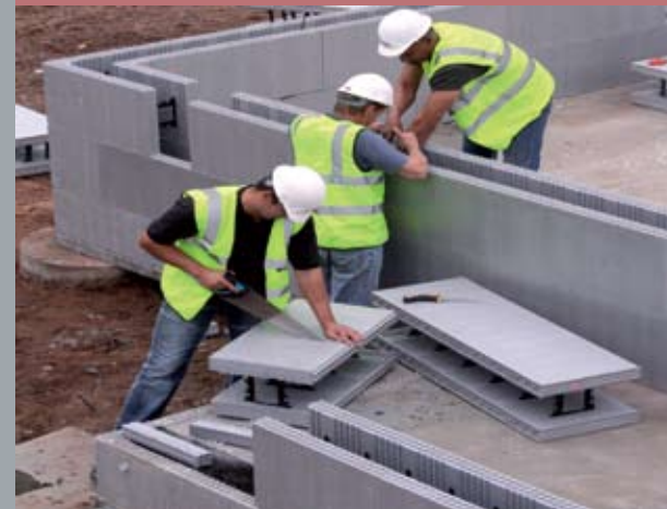
Insulating Concrete Forms (ICFs) offer solid, lasting construction that resists the ravages of fire, wind, and time as well as providing two built-in layers of foam insulation.
