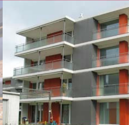
Passive house using Neopor®, Constance (Switzerland) Façade insulation (30 cm)
