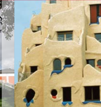
"Les Grottes" insulating plaster façade, Geneva (Switzerland)
