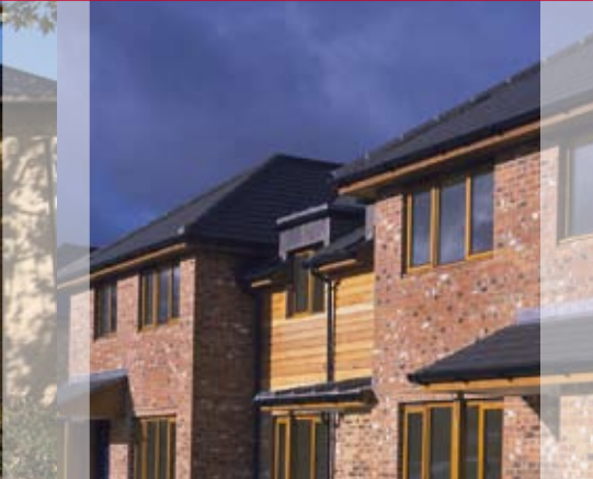
Social housing construction, London (GB) Steel frame design with foamed Neopor® (13 cm)
