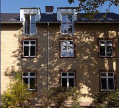
Old building renovation using Neopor®; Ludwigshafen (Germany): roof insulation (40 cm), interior insulation (8 cm) and cellar ceiling insulation (7 to 10 cm)
